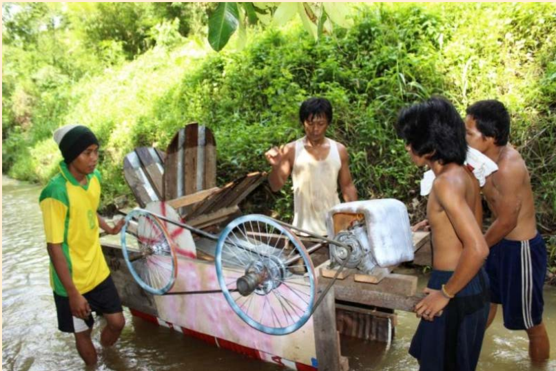
the installation of the hydroelectric power prototype
