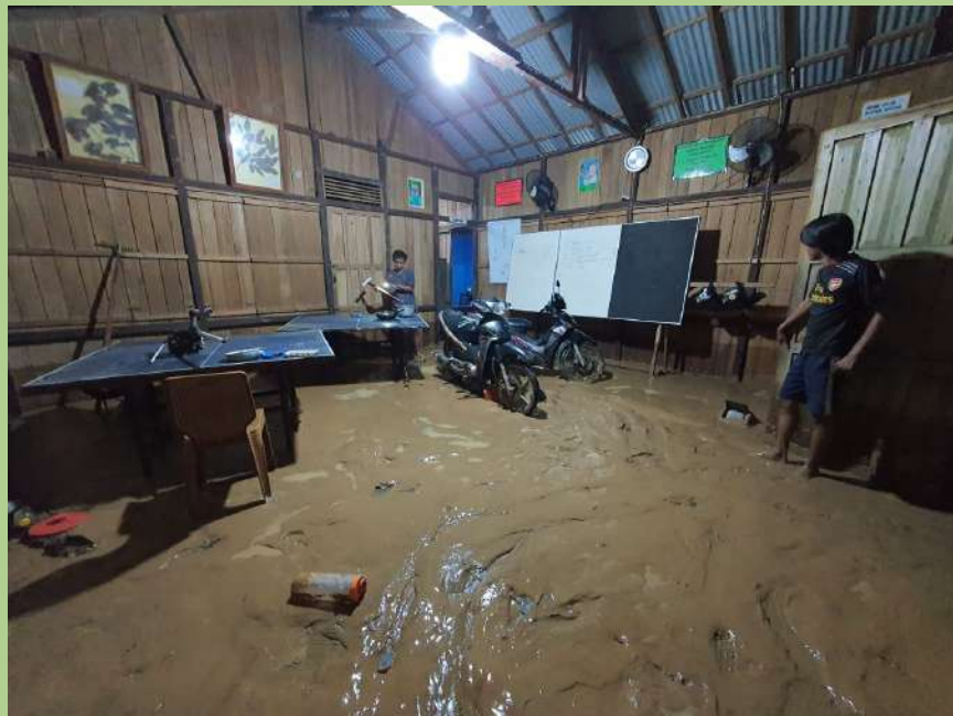
Mud covers the floor inside Bentangor the day after the building flooded.
